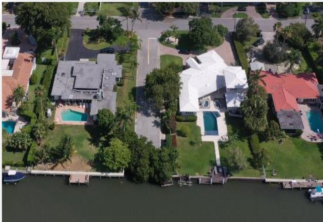
Tidal Flooding Mitigation
