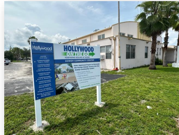
Dowdy Former Armory to become the Dowdy Community Center
